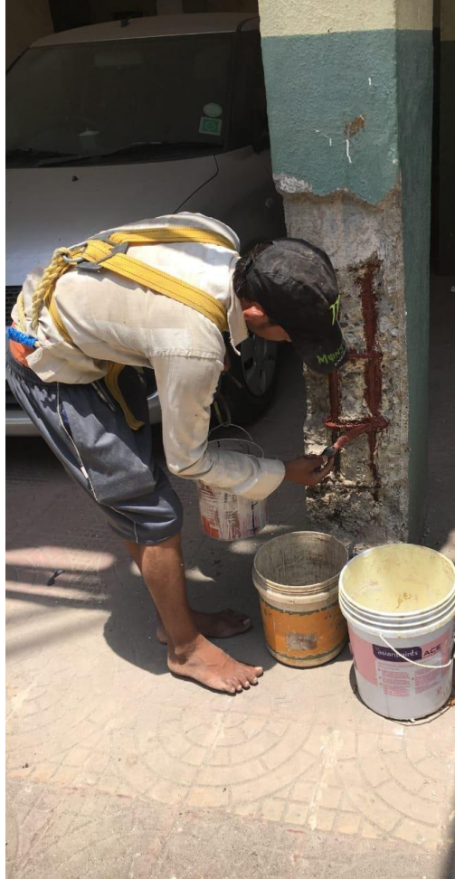
Step-2: Anti corrosion treatment
