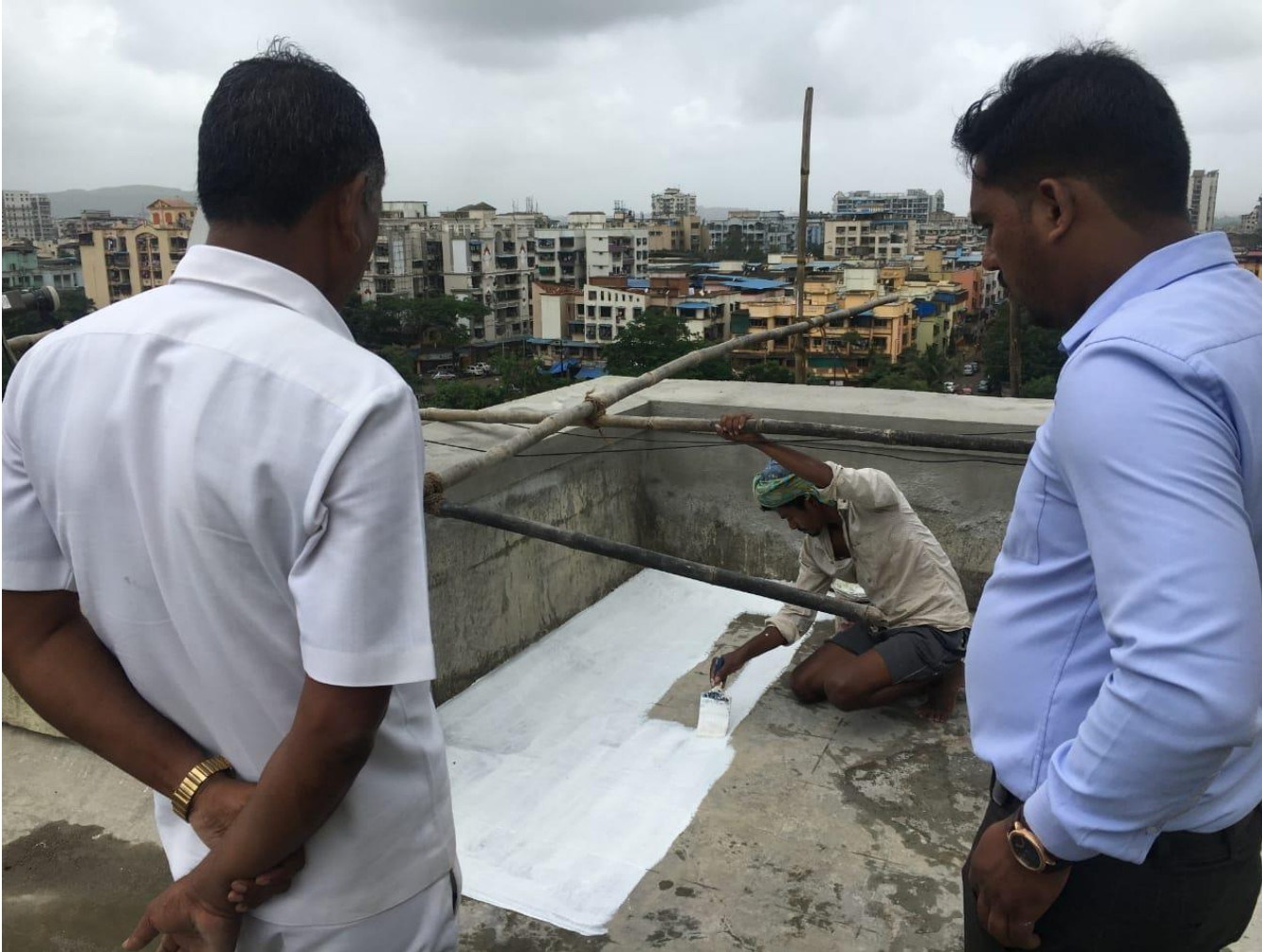
On site personal inspection & supervision by Mr. Gorakh Pisal & Mr. Dattatray Pisal (waterproofing chemical compound coating)
